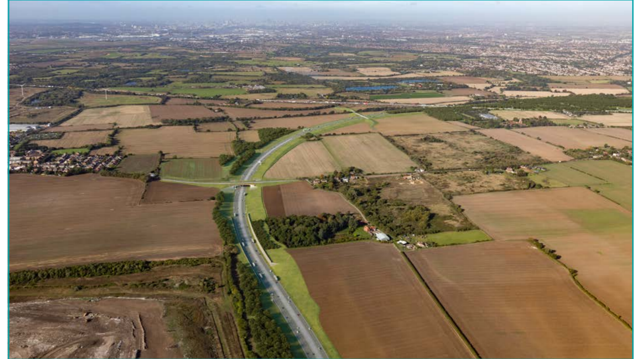
Figure 3-31. Design refinement consultation – proposed North Road green bridge over the LTC, looking west
