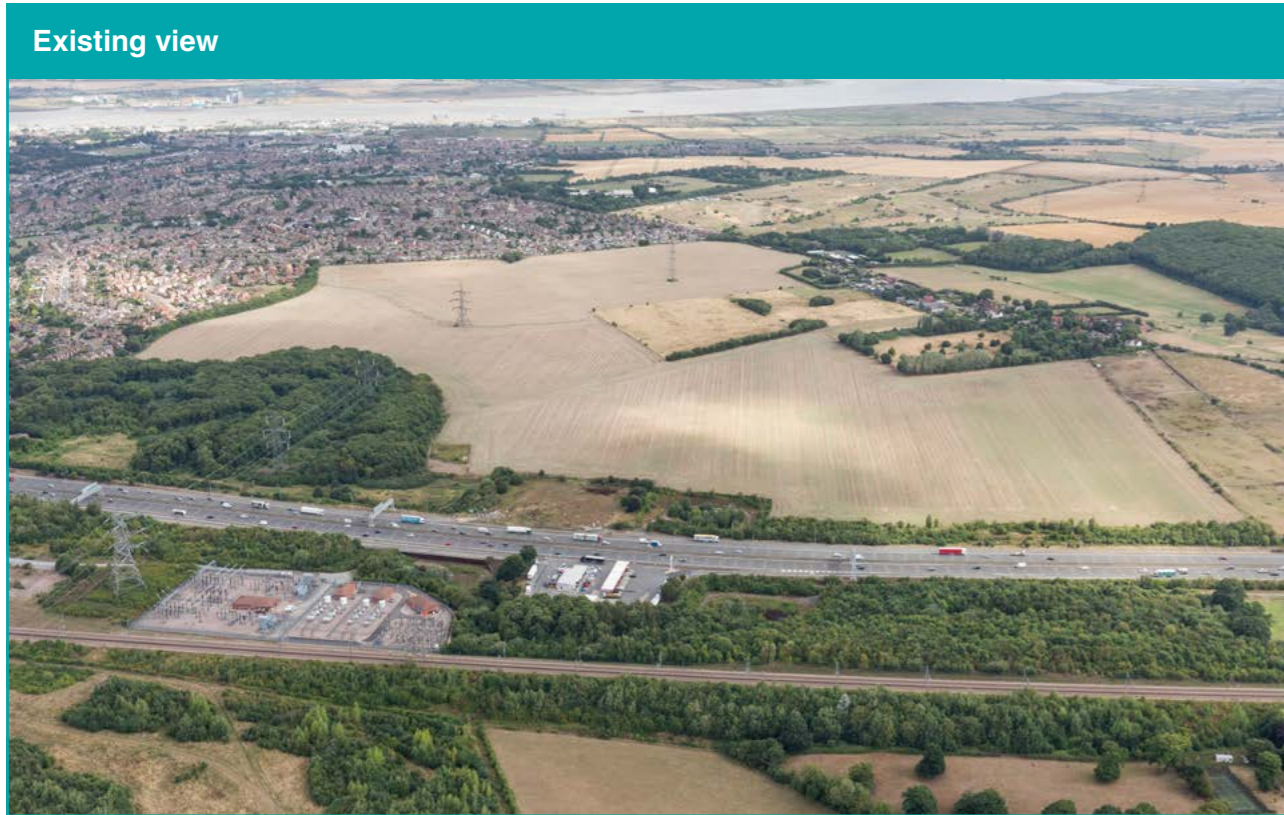
Figure 3-5. Existing A2, looking north
