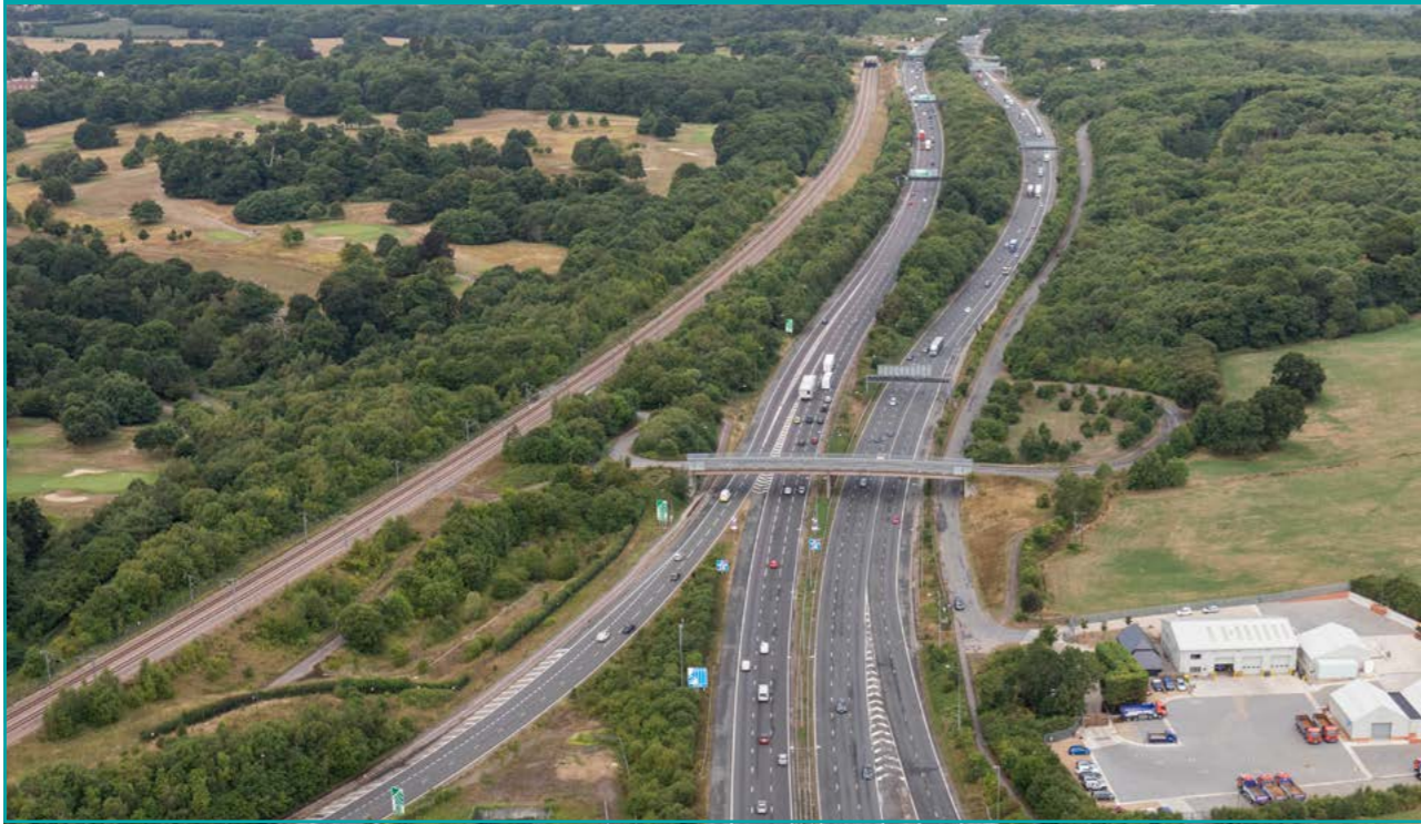
Figure 3-1. Existing M2/A2 along the A2 near Park Pale bridge, looking west
