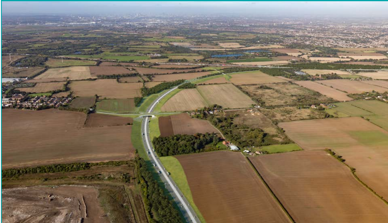
Figure 3-30. Supplementary consultation – proposed North Road green bridge over the LTC, looking west
