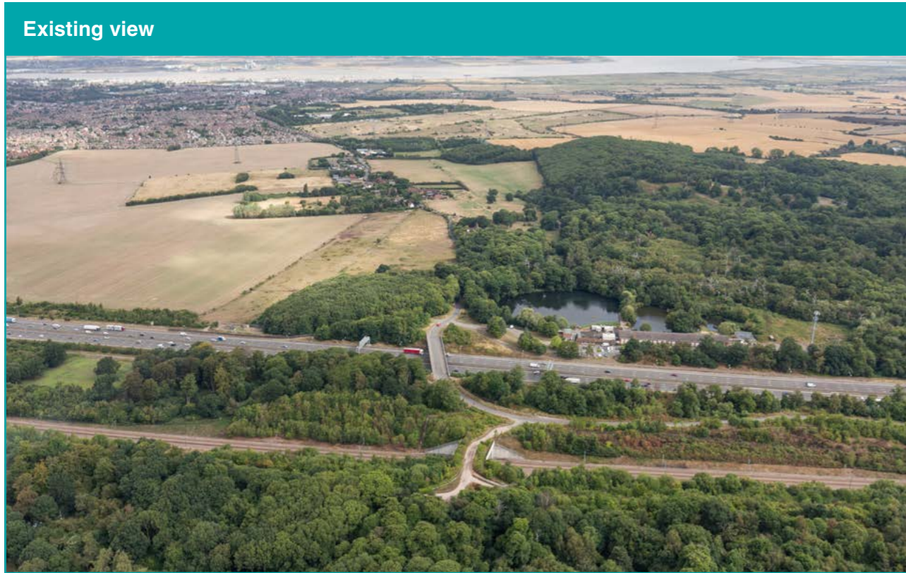
Figure 3-9. Existing Thong Lane and A2, looking north
