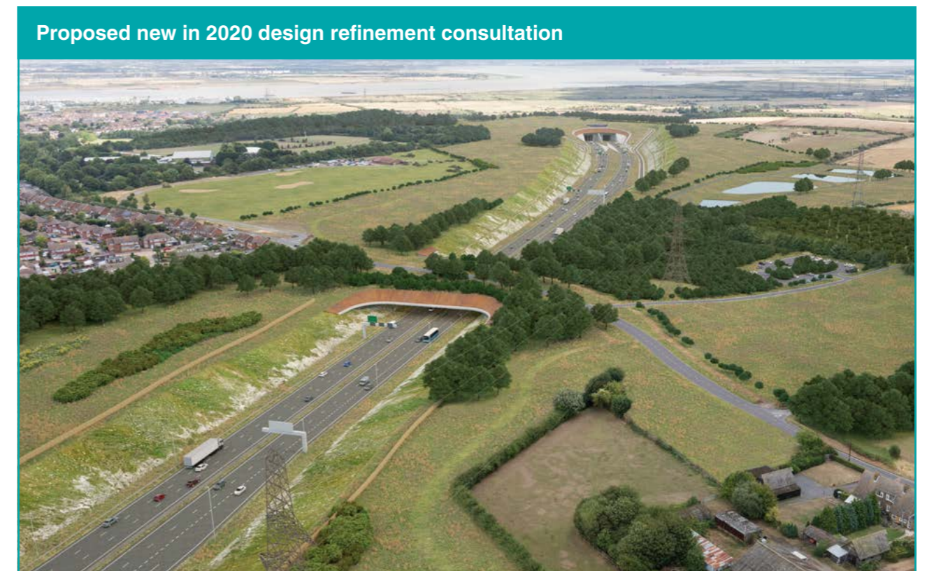
Figure 3-15. Design refinement consultation – proposed Thong Lane green bridge linking Gravesend and Thong and the approach to the southern tunnel entrance, looking north
