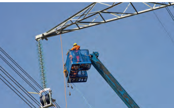
Example of pylon stringing
