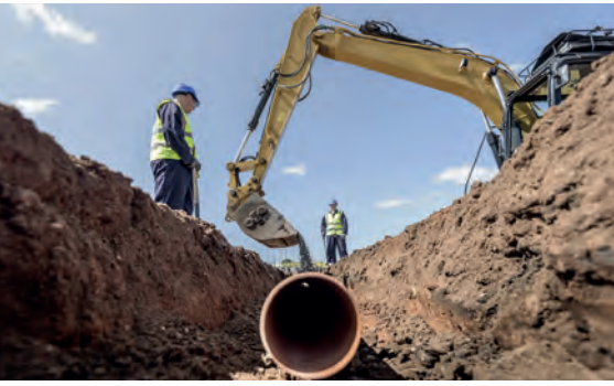
Example of an open-cut trench technique
