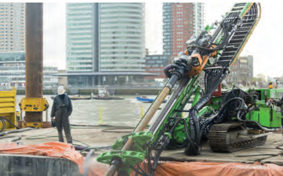
Example of an HDD trenchless technique
