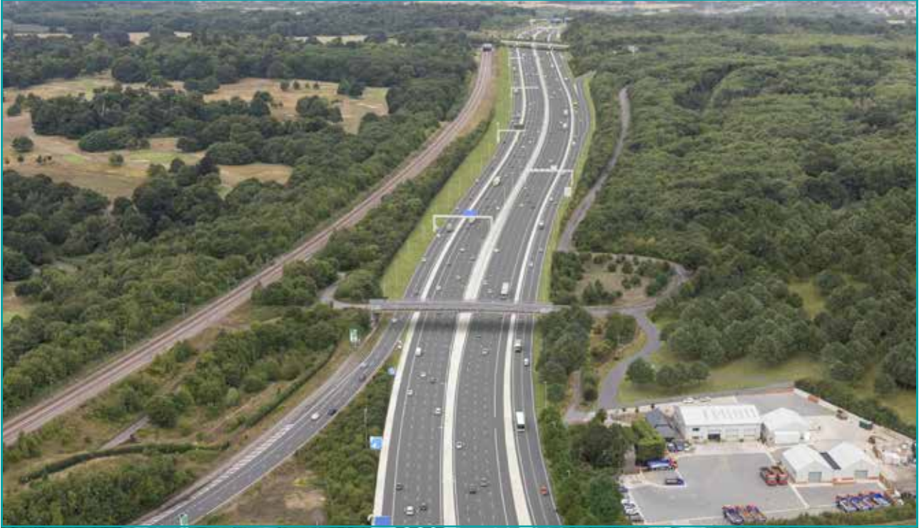
Figure 5-13. Supplementary consultation – proposed M2/A2 along the A2 near Park Pale bridge, looking west
