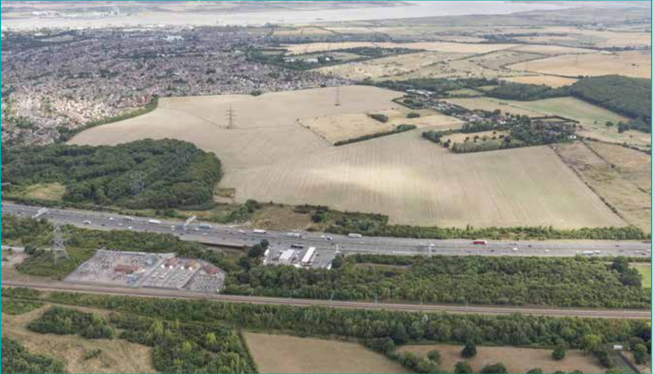
Figure 5-14. Existing A2, looking north
