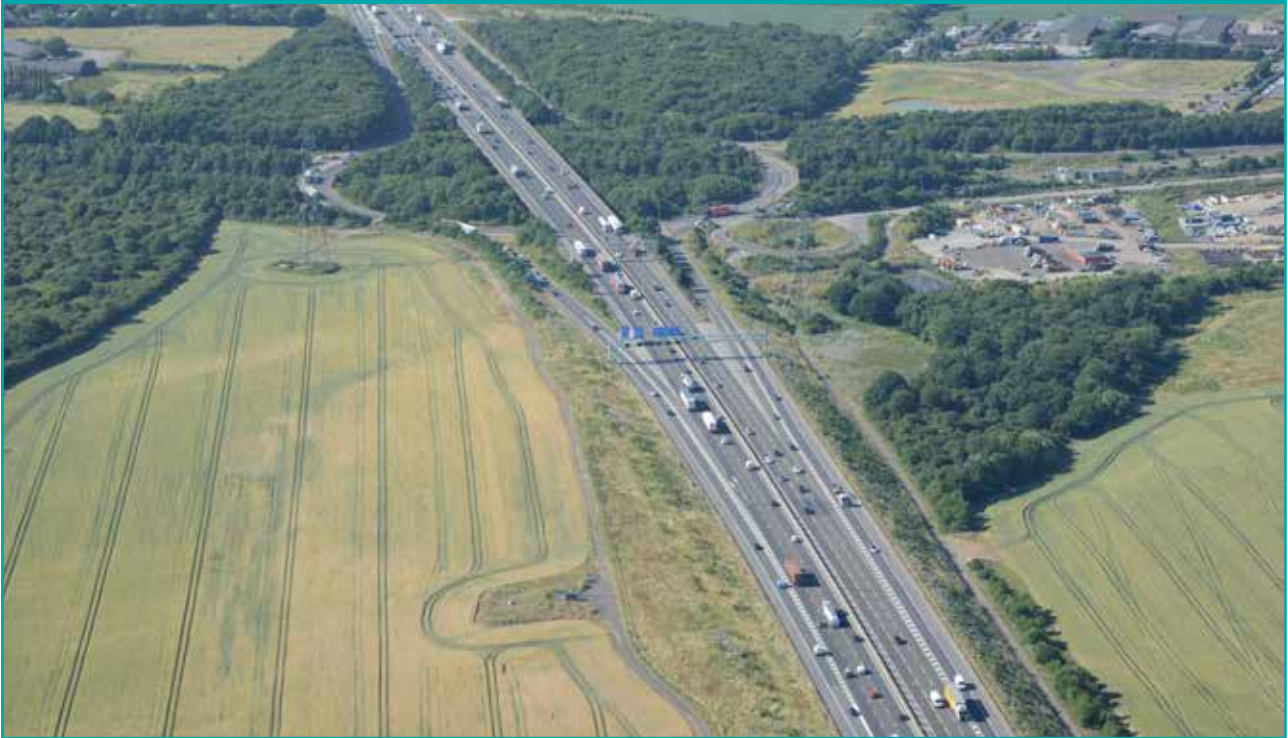
Figure 5-59. Existing view of M25 between junction 29 and 30, looking north
