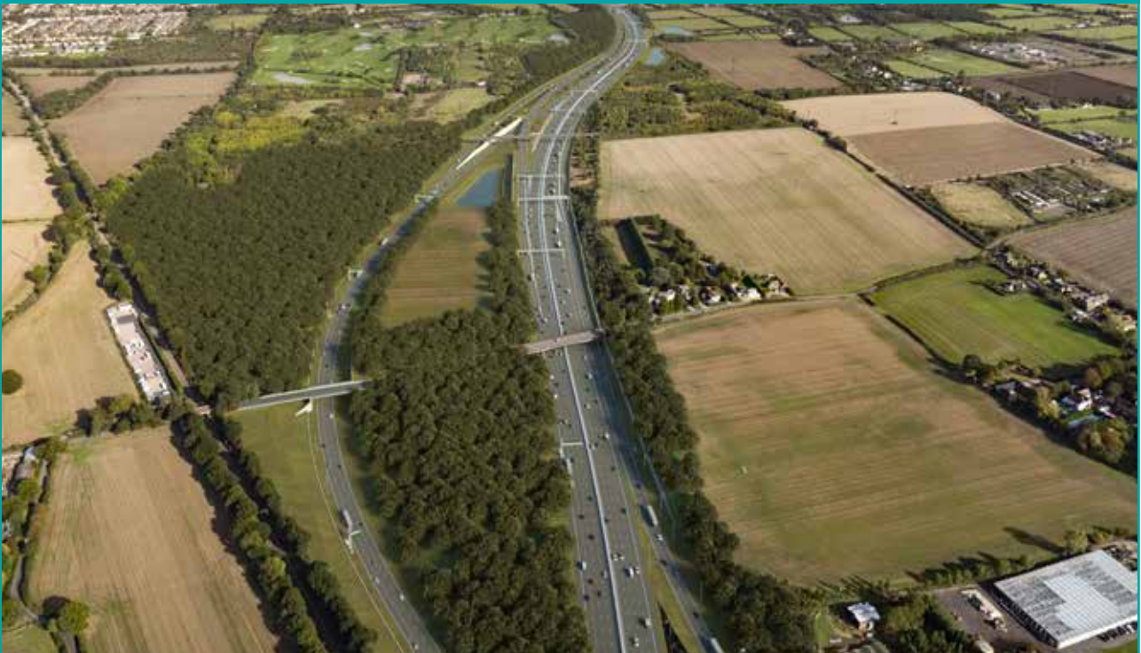
Figure 5-58. Supplementary consultation – proposed LTC/M25 junction, with new Ockendon Road bridge, looking north
