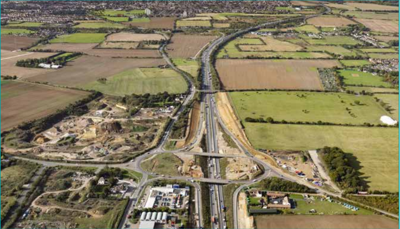
Figure 5-46. Existing A13/A1089 junction at the Orsett Cock roundabout, looking west
