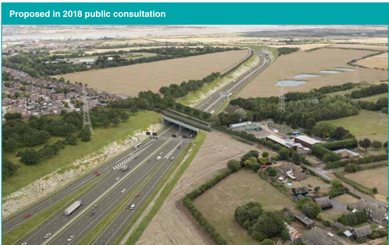
Figure 5-22. Statutory consultation – proposed Thong Lane bridge linking Gravesend and Thong, and the approach to the south tunnel entrance, looking north
