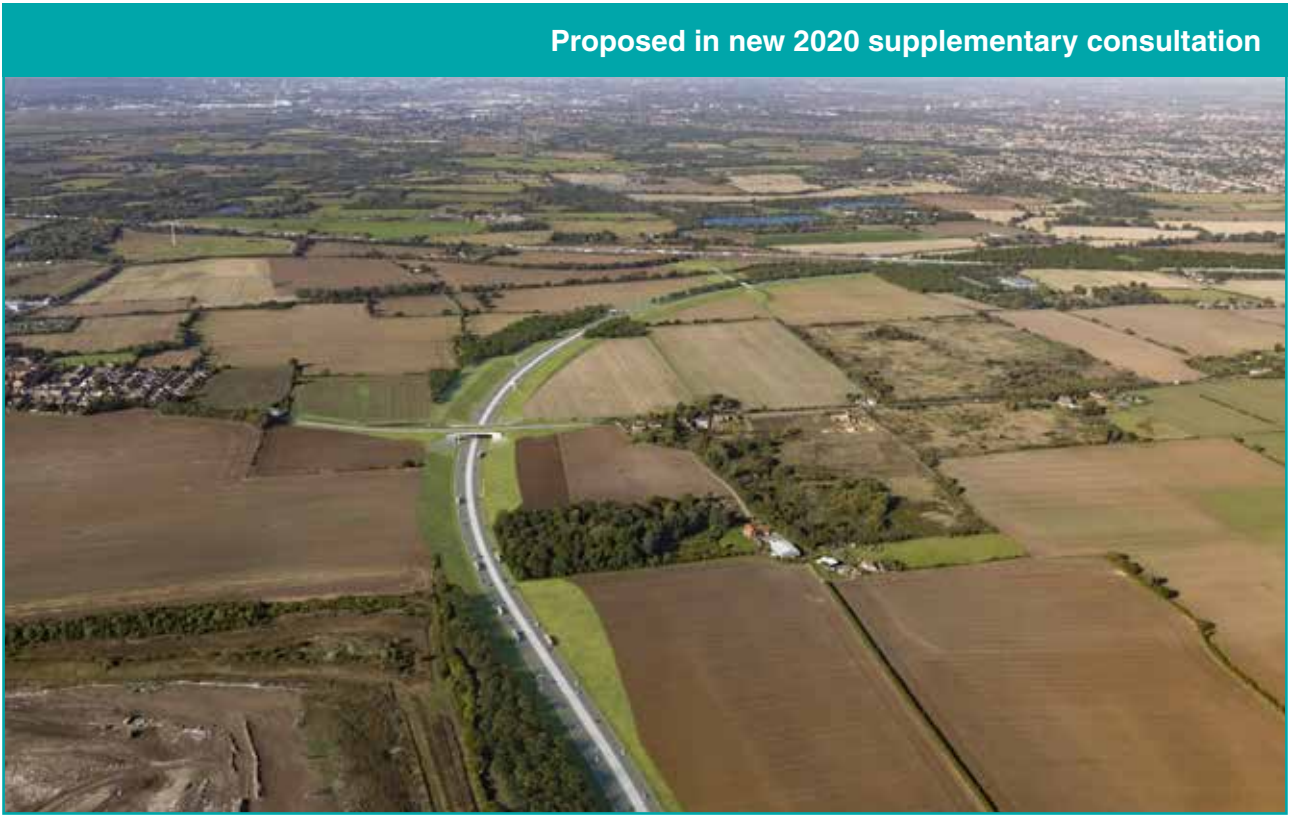
Figure 5-56. Supplementary consultation – proposed North Road green bridge over the LTC, looking west
