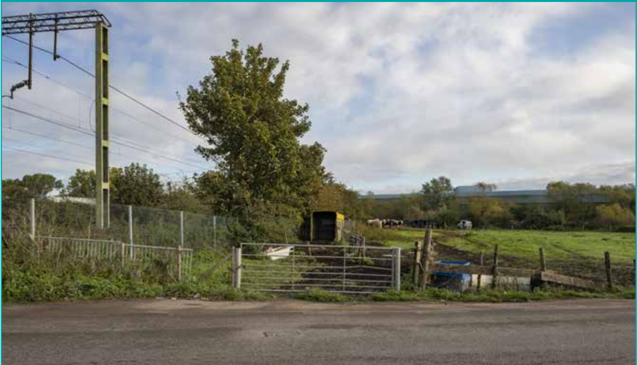
Figure 5-37. Supplementary consultation – proposed Tilbury viaduct from properties on Station Road, looking north-east
