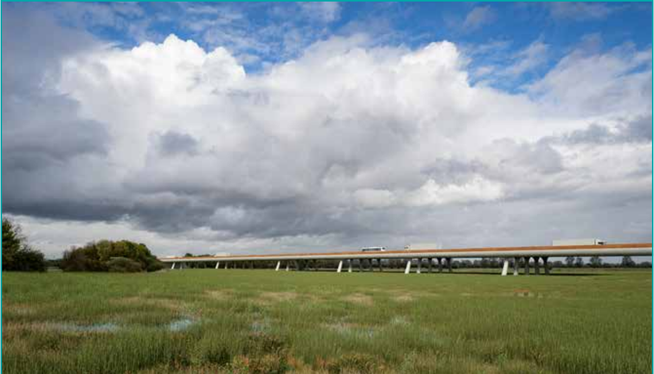
Figure 5-54. Supplementary consultation – proposed Mardyke viaduct and wetland creation, from the Mardyke trail, looking north
