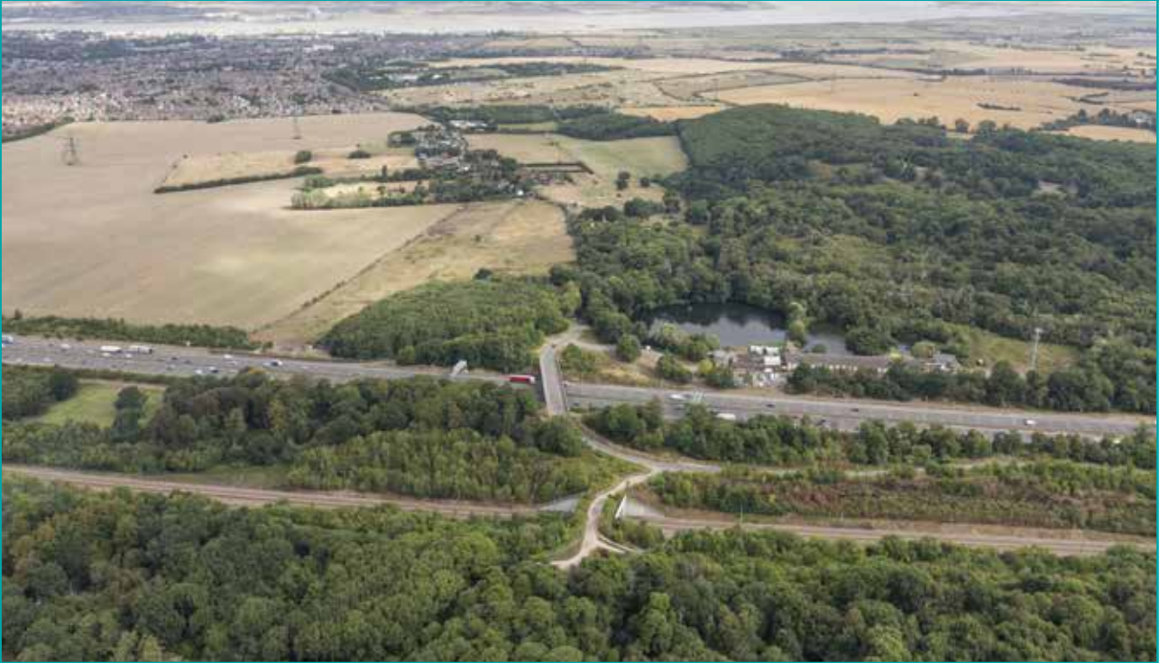
Figure 5-17. Existing Thong Lane and A2, looking north
