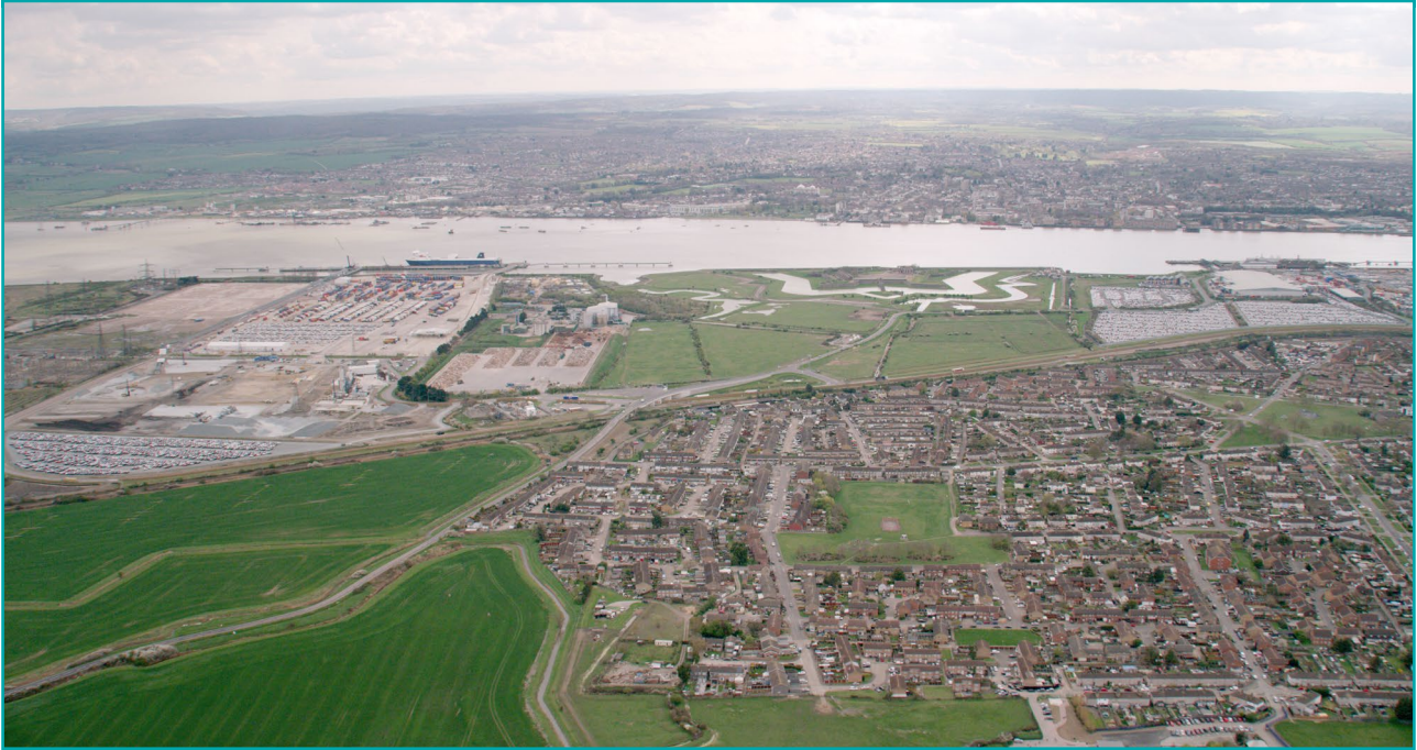
Figure 3-13 Current view of Port of Tilbury infrastructure corridor looking south
