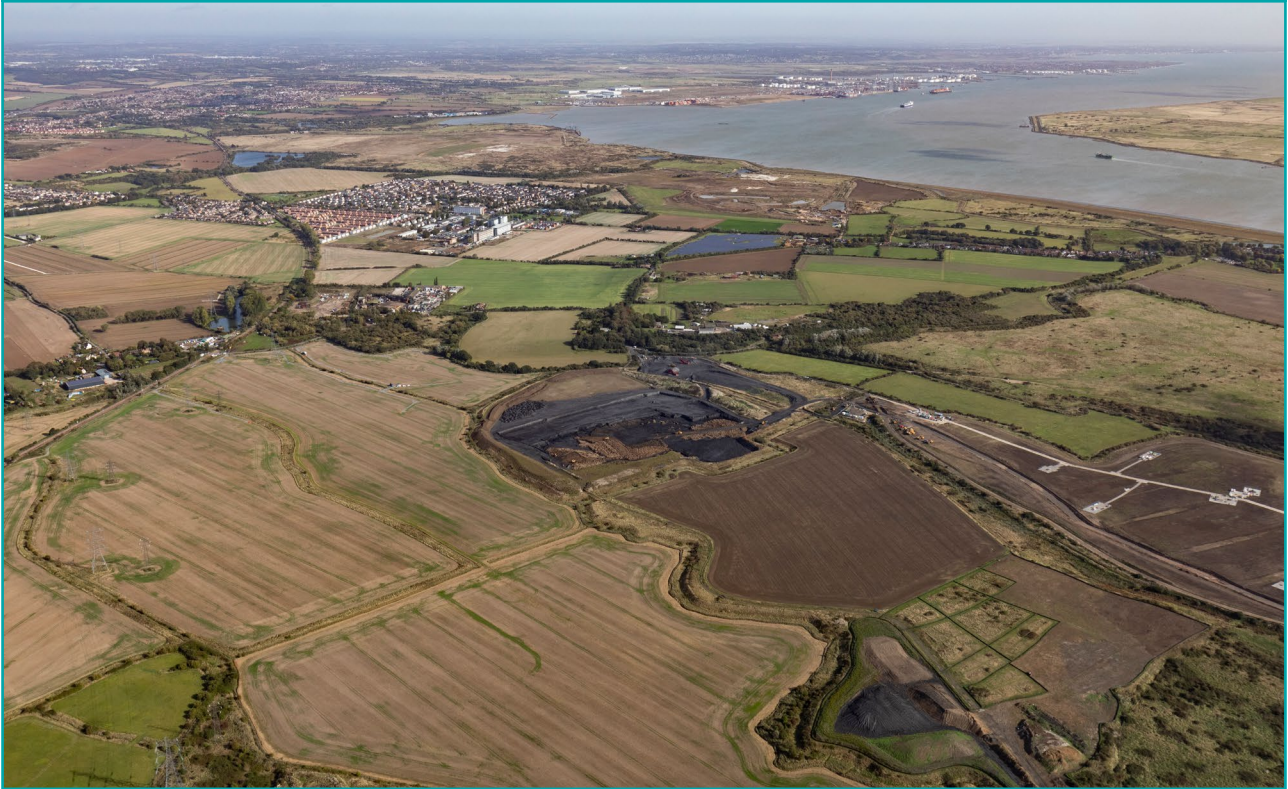
Figure 3-14 Current view of Tilbury area looking east
