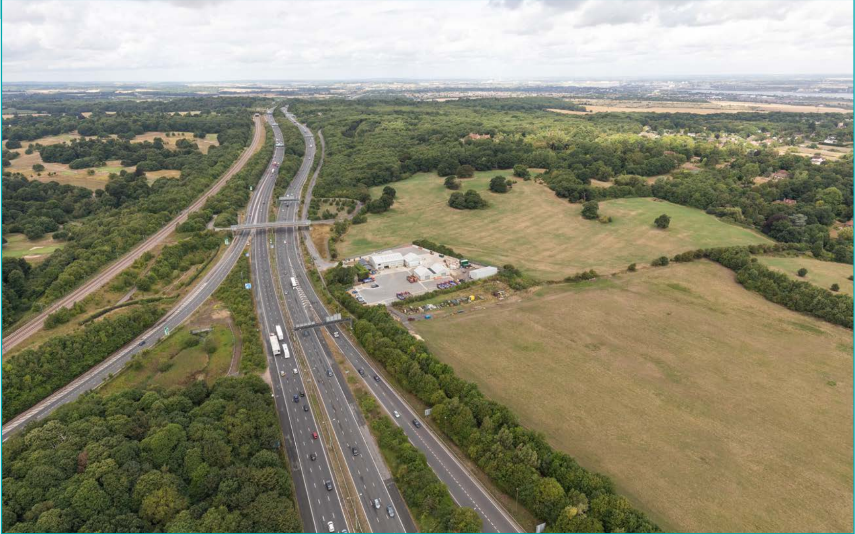
Figure 8-1 Existing view of the A2 corridor from east of Brewers Road, looking west
