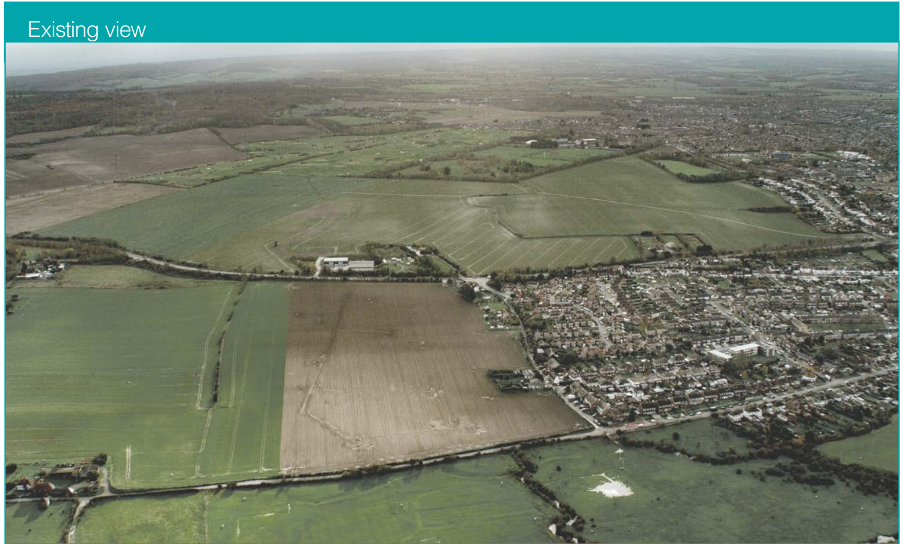
Figure 8-7 Existing view of the South Tunnel Entrance Compound site from south of Chalk, looking north
