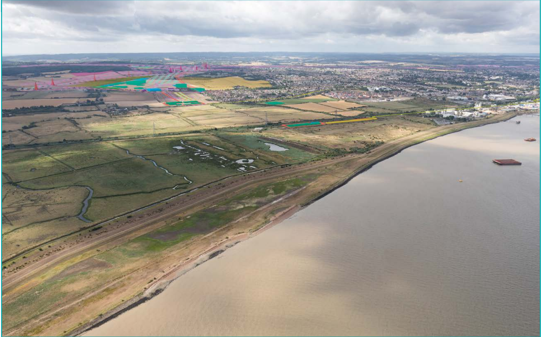
Figure 8-12 Indicative view during construction of Shorne Marshes from the River Thames, looking south-west, showing the A226 Gravesend Road Compound, Milton Compound and combined utilities and highway/tunnel construction areas
