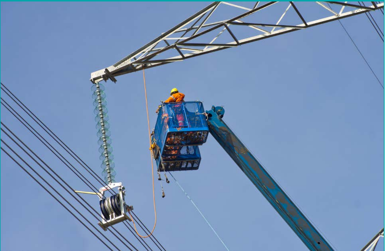
Figure 2-8 Electrical worker building an electricity pylon
