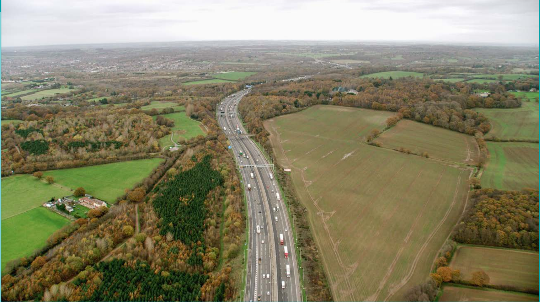
Figure 8-35 Existing view of the M25 corridor and Folkes Lane Bridge from the south, looking north
