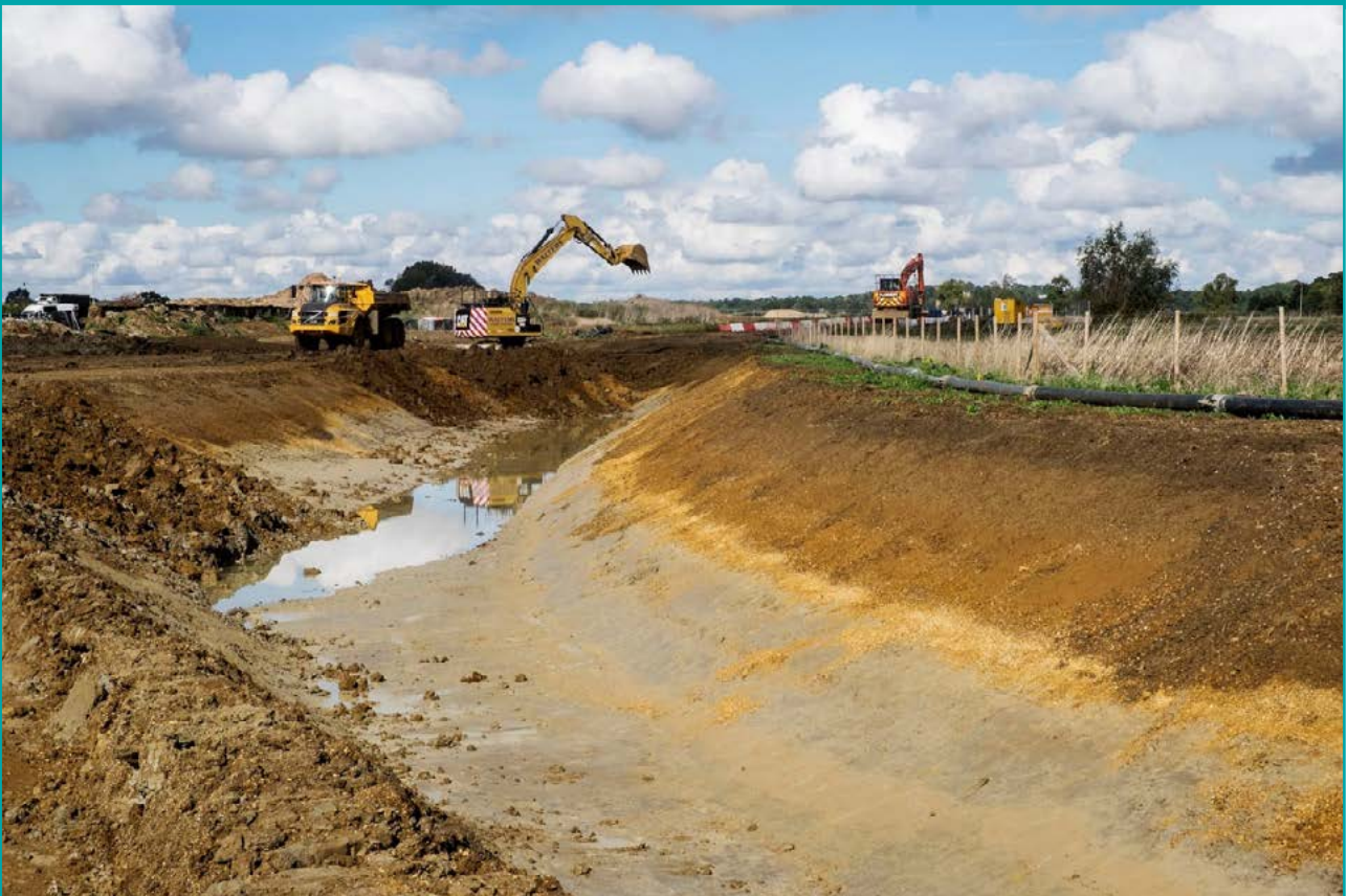
Figure 2-6 A digger being used to excavate a cutting
