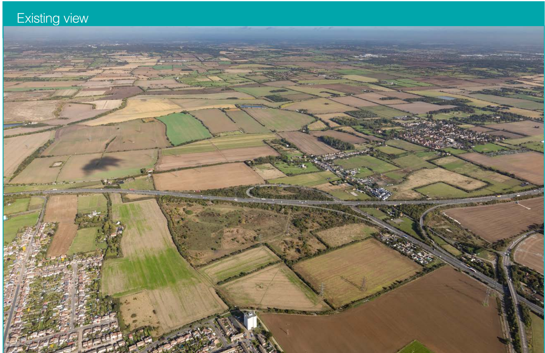
Figure 8-23 Existing view of the A13 junction and Blackshots Nature Reserve from the south-west, looking north towards Baker Street and Orsett
