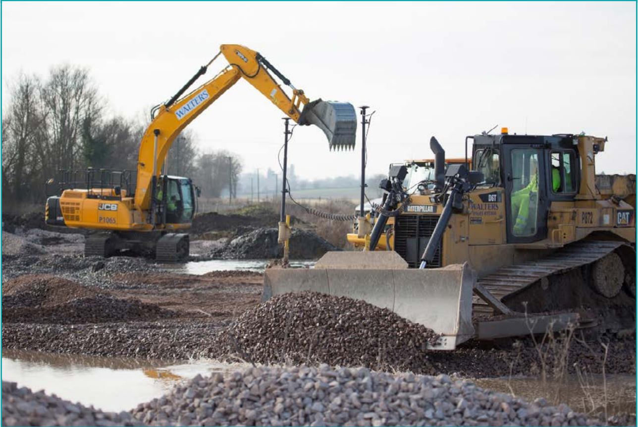
Figure 2-1 Construction machinery moving aggregate into place
