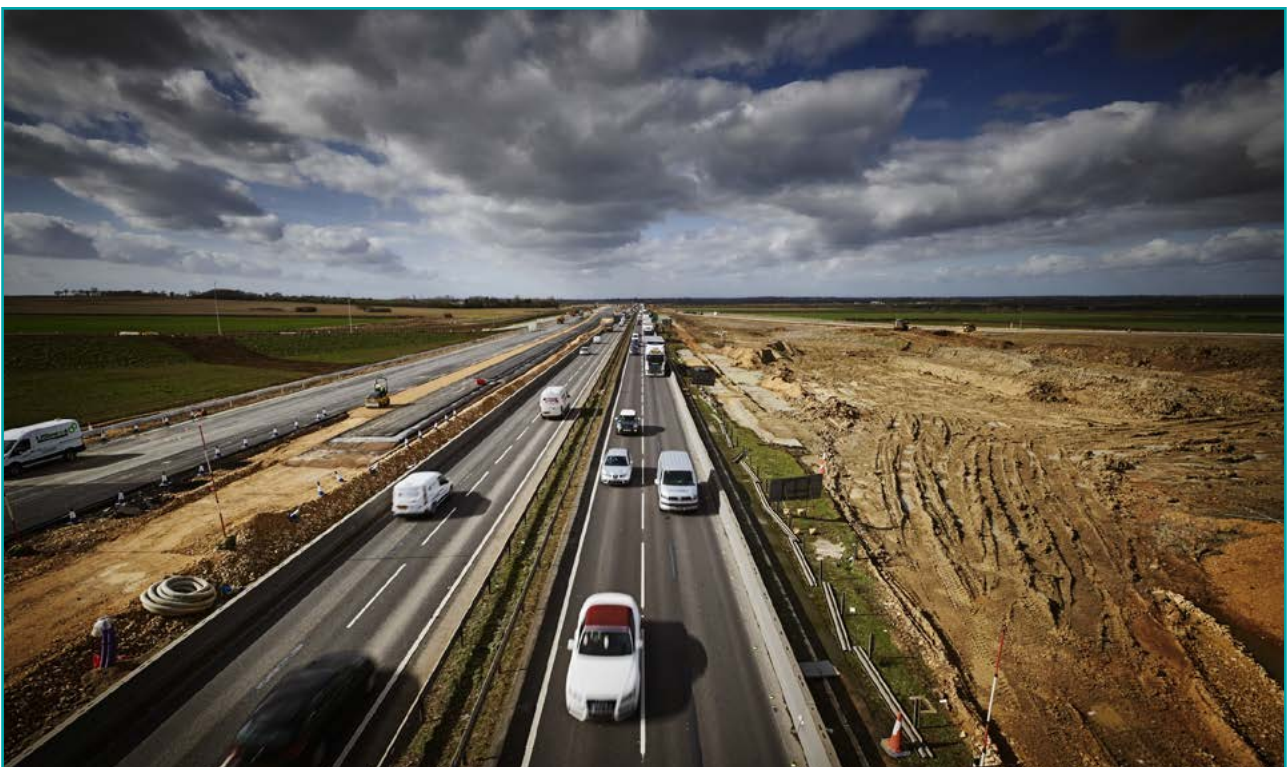
Figure 2-2 Ground beside carriageway prepared for works and new carriageway under construction
