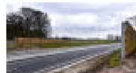
A typical noise barrier
