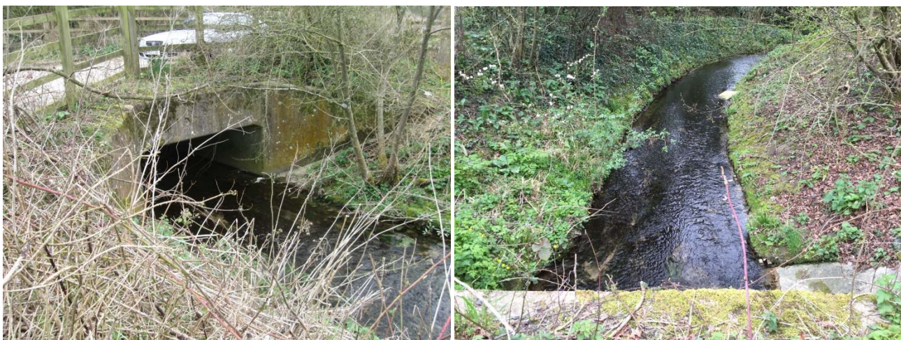
Figure 13.5 - East Stour River (left: culvert after M20, right: from culvert towards CTRL)
