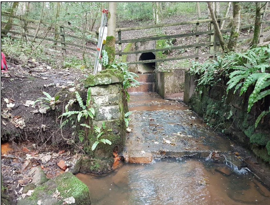
Plate C8: View towards Bradley Brook culvert outlet from M60 (looking upstream). Concrete cascade feature enters from the right (left bank) behind fence line.
