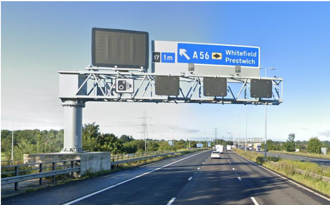
Plate 2.1: A sign and signal long span cantilever gantry on the M60
