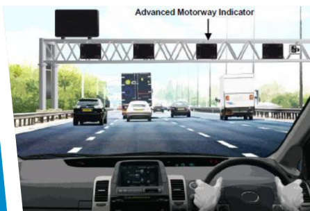
Figure 4c: Illustrative smart motorway All lane running scheme section operating with variable mandatory speed limits.
