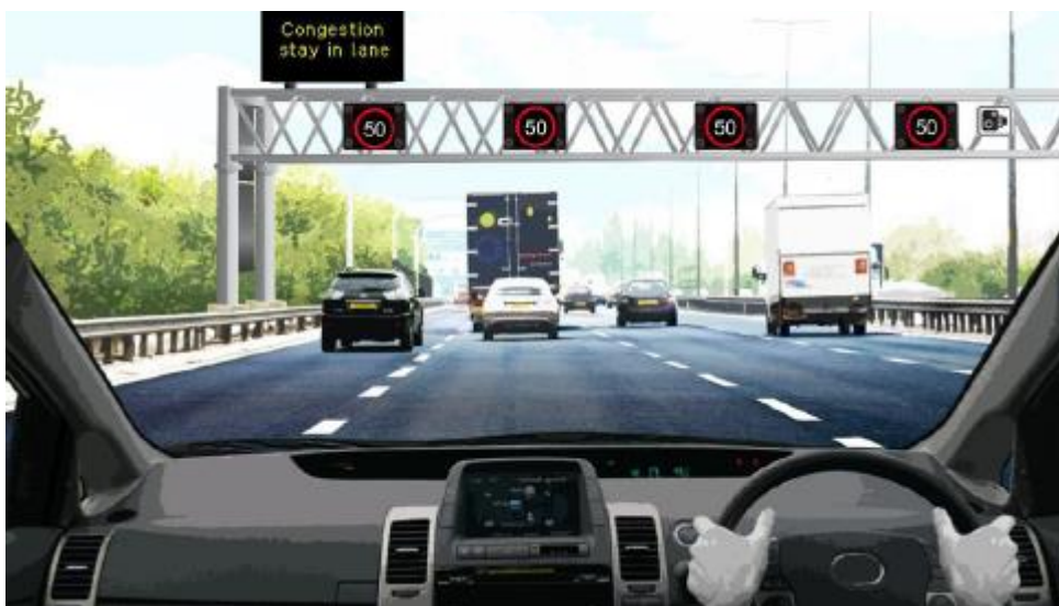
Figure 4c: Illustrative smart motorway all-lane running scheme section operating with variable mandatory speed limits due to congestion
