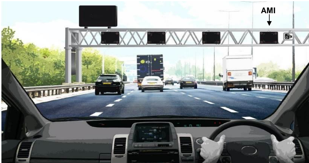
Figure 4A: Illustrative M6 J2 to J4 smart motorway scheme section operating in normal motorway conditions with blank AMI and blank gantry mounted VMS
