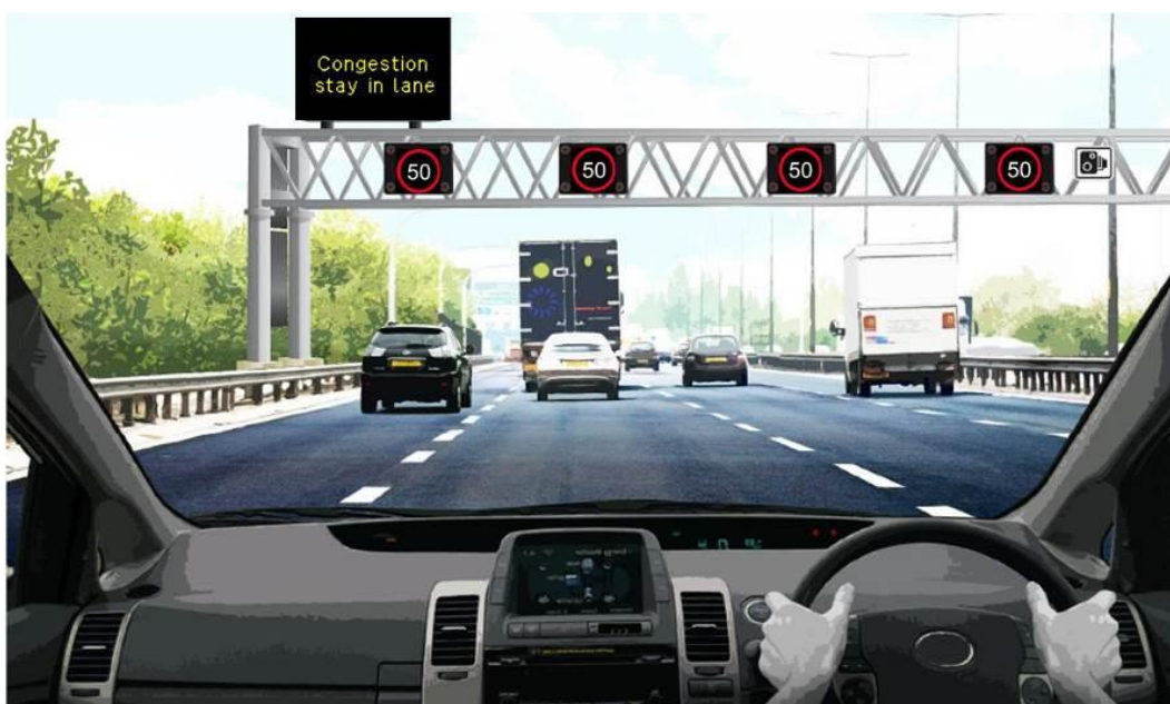
Figure 4C: Illustrative M6 J2 to J4 smart motorway scheme section operating with variable mandatory speed limits
