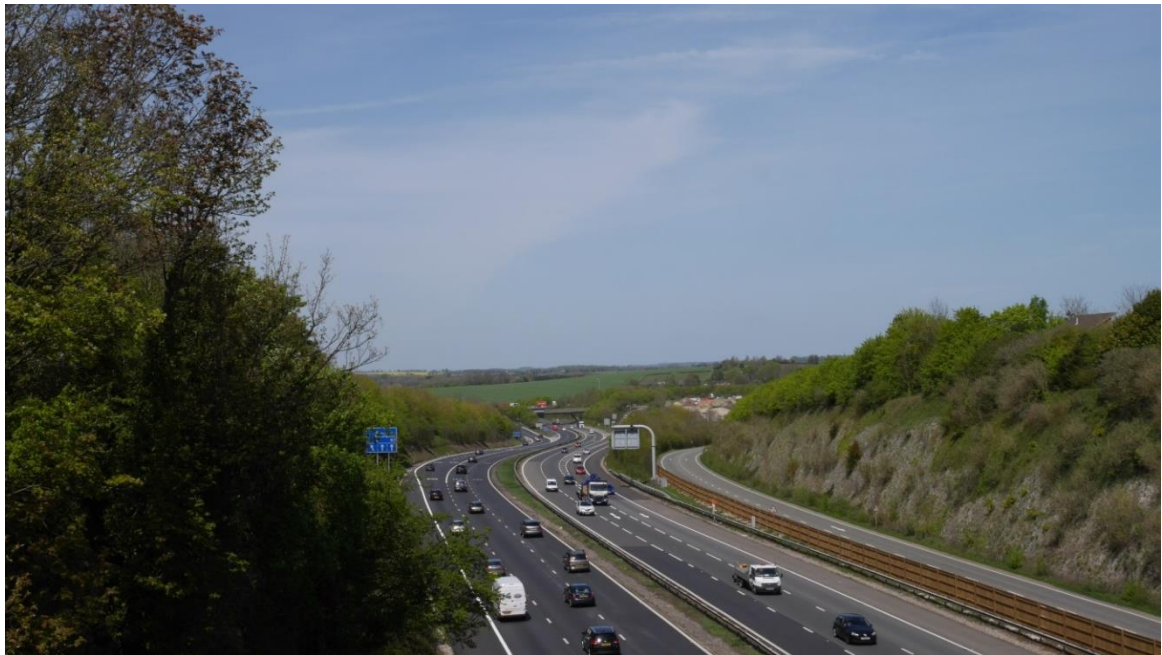
Figure 7-13: Viewing north from the B3404 roadbridge
