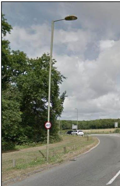
Figure 4-14: Windhover Roundabout Asset
