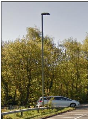
Figure 4-16: M27 Junction 8 Asset
