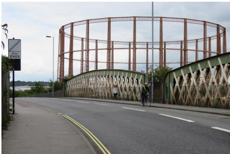
Figure 9-7: Northam Rail Bridge
