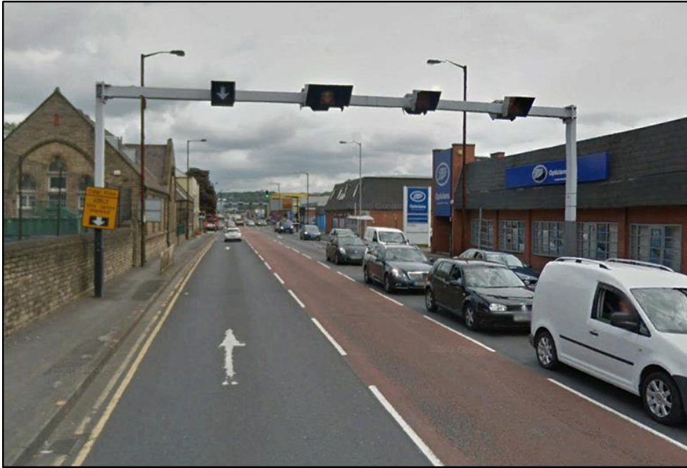
Figure 18-2: Example of Tidal Flow arrangement in Sheffield (#2)
