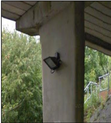
Figure 4-17: M27 Junction 8 Asset
