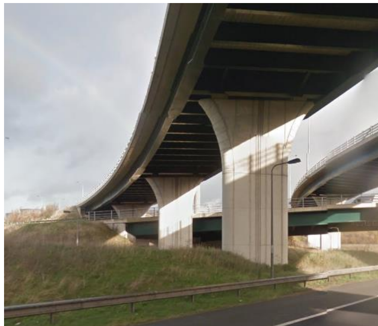
Figure 2: Proposed tapered pier form for steel composite ladder beam deck
