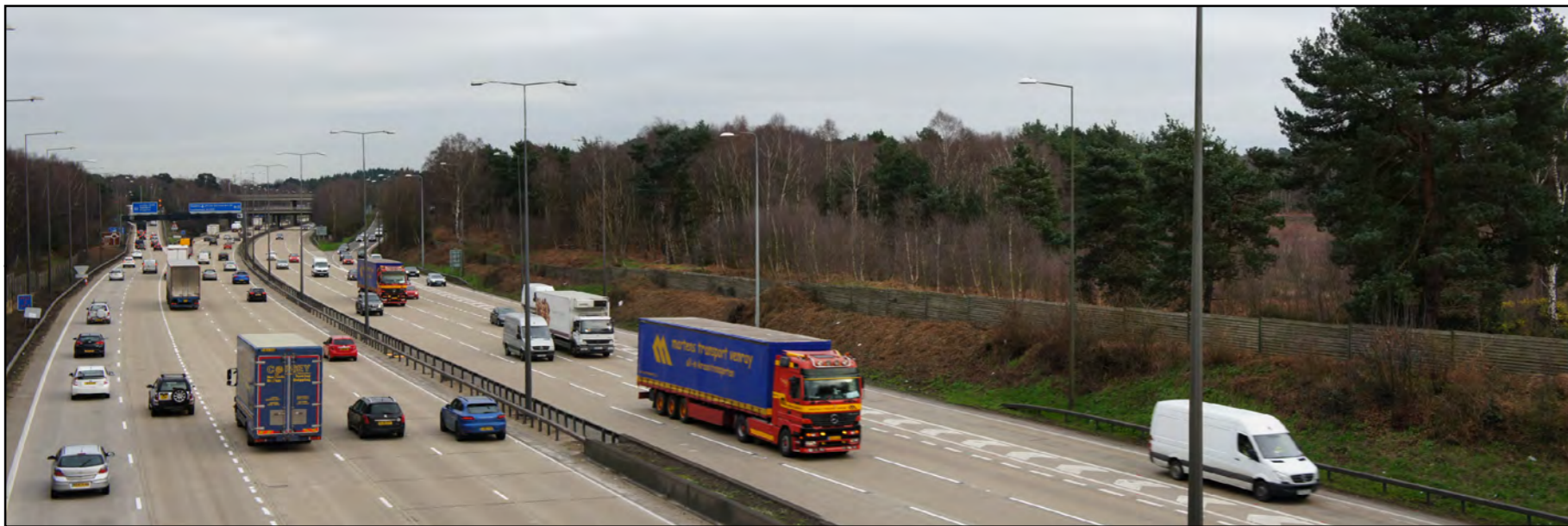
Viewpoint 9: View from Footpath 17 (overbridge) looking north
