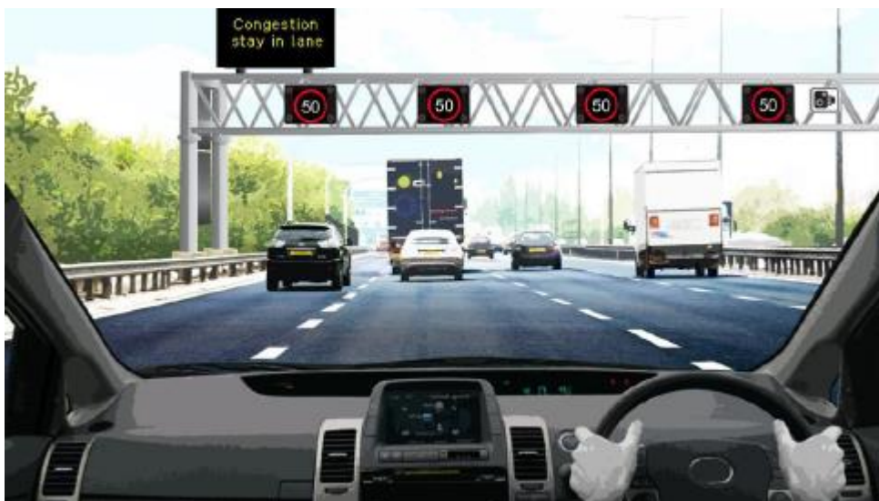
Figure 4c: Illustrative smart motorway all-lane running scheme section operating with variable mandatory speed limits
