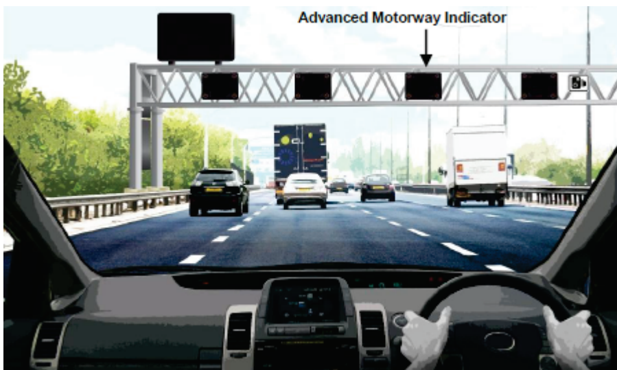
Figure 4a: Illustrative smart motorway all-lane running scheme section operating in normal motorway conditions with blank advanced motorway indicators and blank gantry mounted variable message sign
