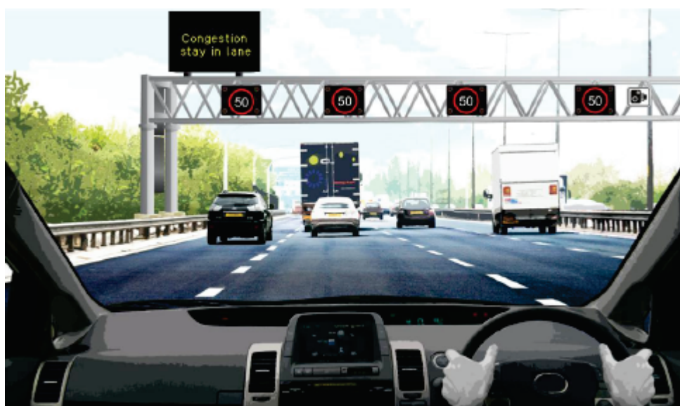
Figure 4c: Illustrative smart motorway all-lane running scheme section operating with variable mandatory speed limits
