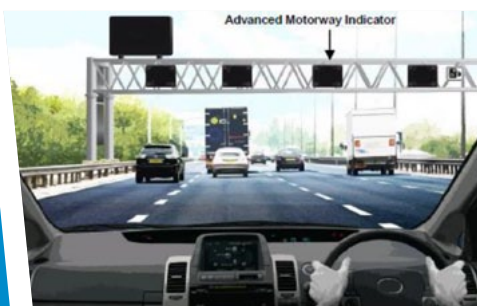
Figure 4c: Illustrative smart motorway All-Lane Running scheme section operating with variable mandatory speed limits.
