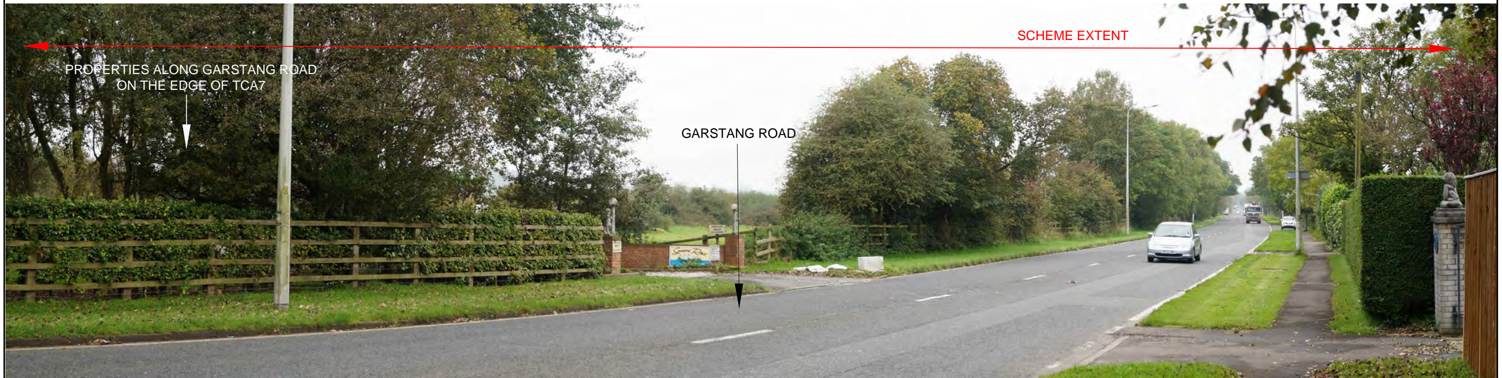
SUMMER VIEWPOINT 14: (A-VP1) VIEW FROM THE A586 GARSTANG ROAD ADJACENT TO RESIDENTIAL PROPERTIES, LOOKING WEST.
