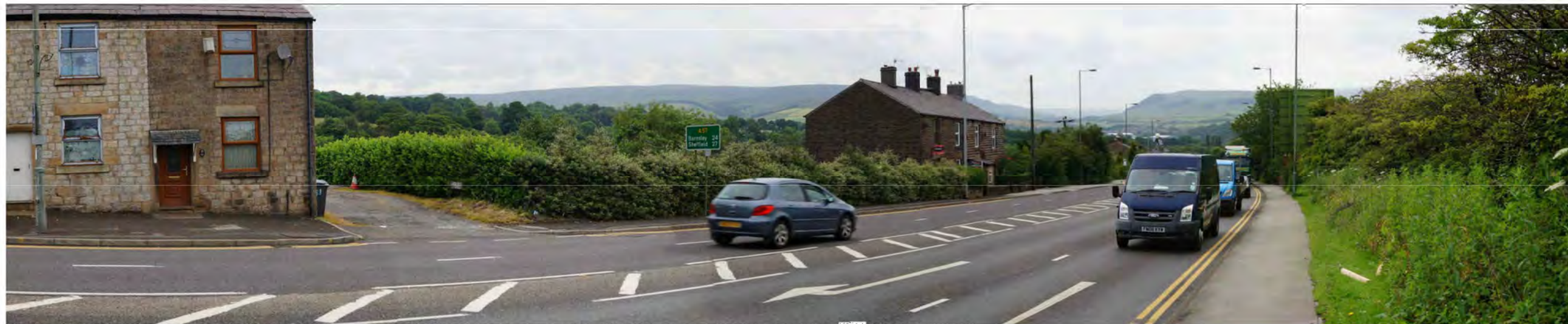
PHOTO VIEW 4; FULL PANORAMIC VIEW - MOTTRAM MOOR LINK ROAD AND A57 (T) TO A57 LINK ROAD, VIEW FROM A57, LOOKING NORTH EAST
