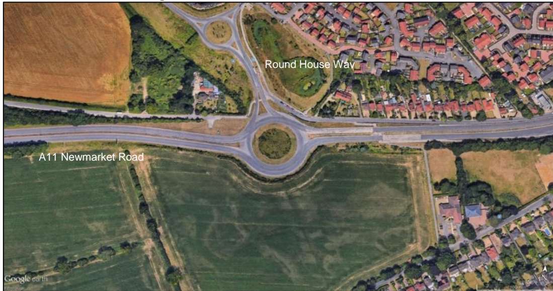
Figure 3-12 Round House Roundabout
