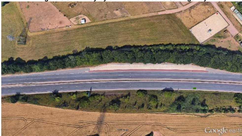
Figure 3-9 Lay-by on A47 Eastbound Carriageway
