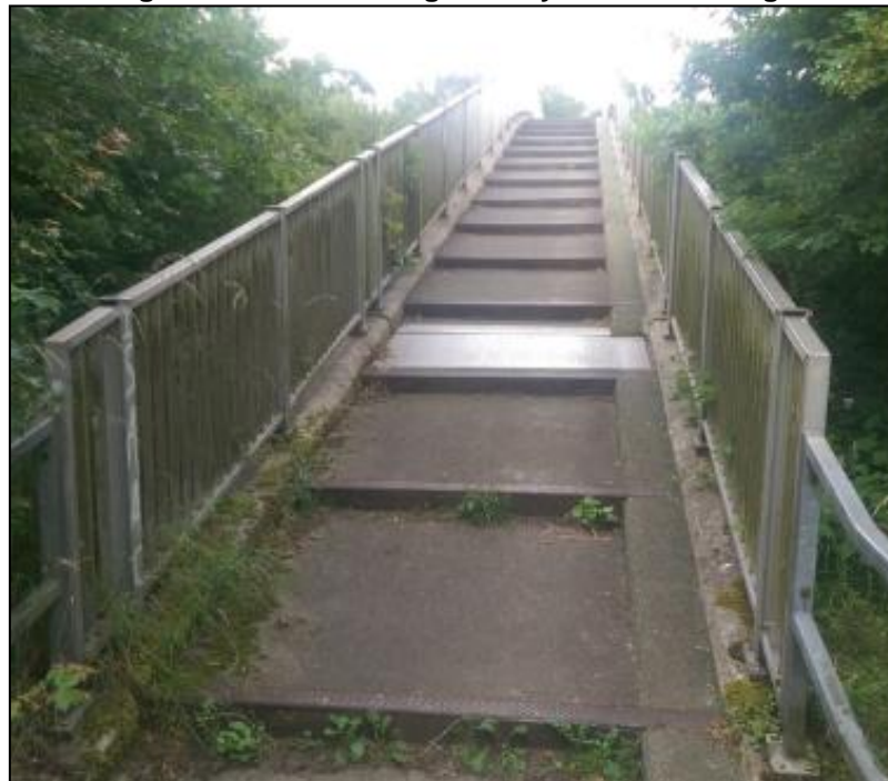
Figure 7-5 Existing Cantley Lane Footbridge
