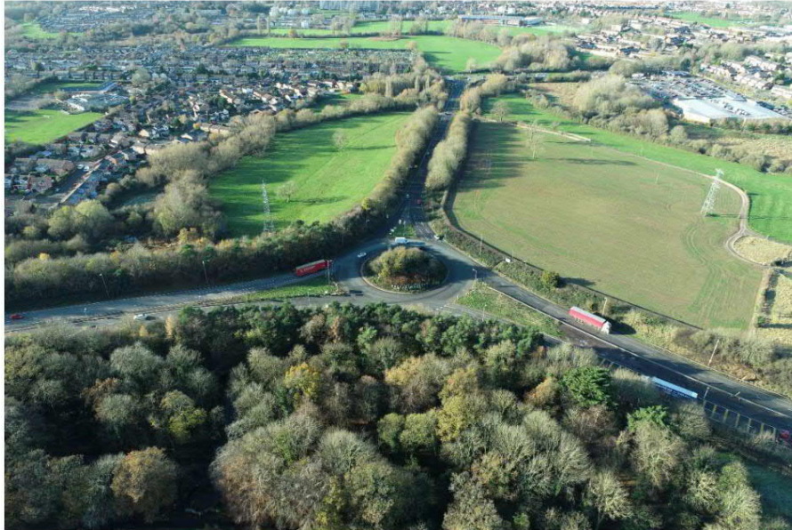
Caption: The existing Walsgrave junction as seen from above.
