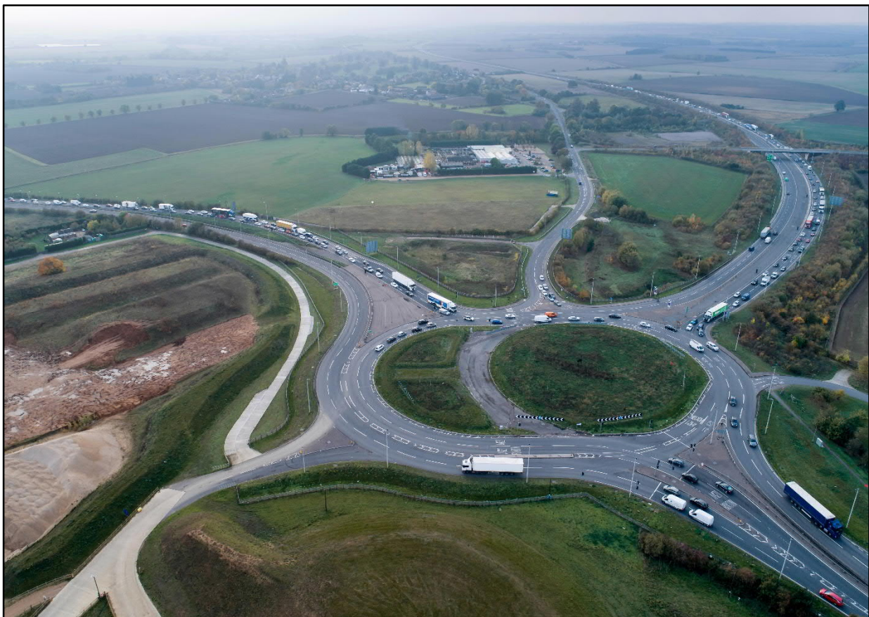
The existing Black Cat roundabout
