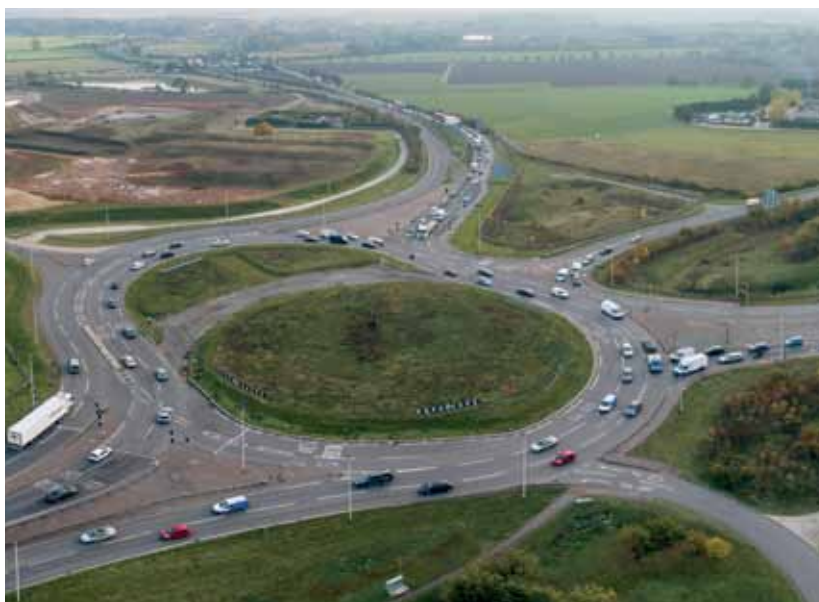
The Black Cat roundabout today (above) and in the future (right).
