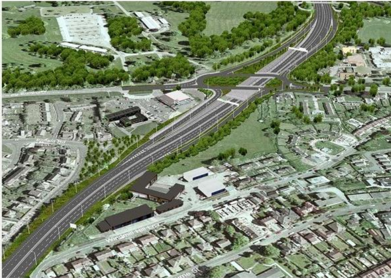
An artist's impression showing the proposed underpass where the Markeaton A38 Island currently sits.
