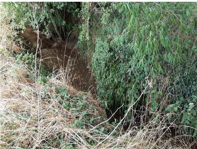
Figure E-36 Site 39 downstream reach
