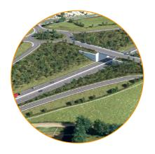
A **cutting** is where the land has been dug into to let the road pass at a lower level than ground level.
