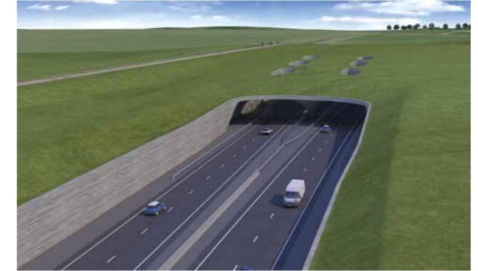
Figure 5.33: Grassed over canopy with ventilation outlets
