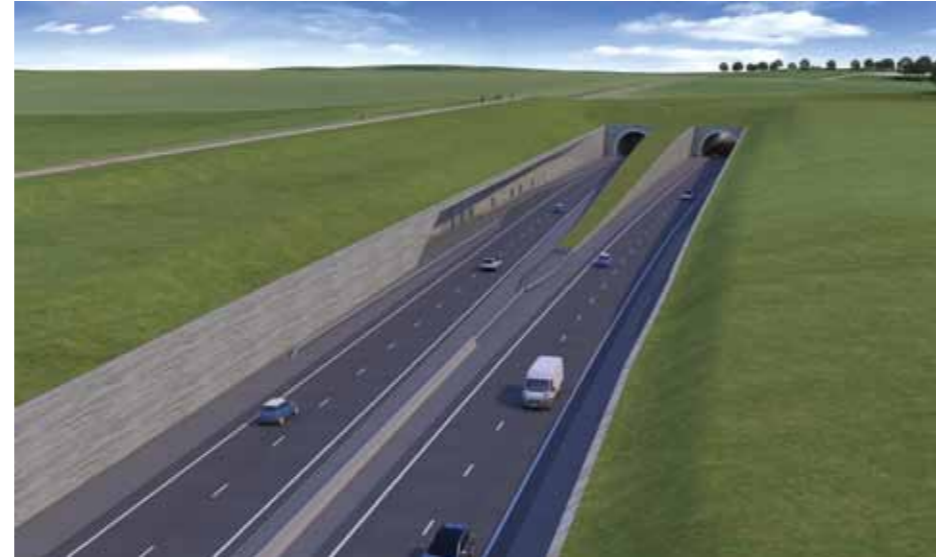
Figure 5.26: Western tunnel entrance - vertical retaining walls option
