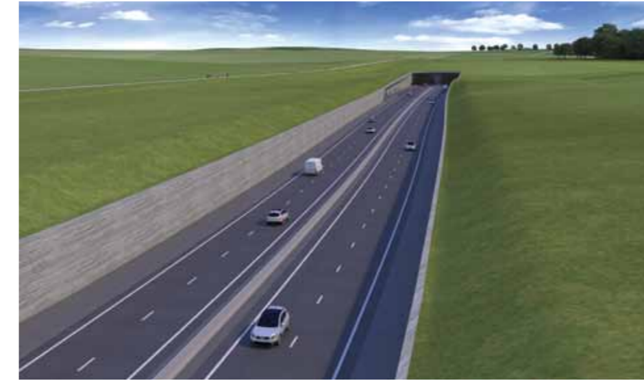
Figure 5.22: Approach option with vertical retaining walls
