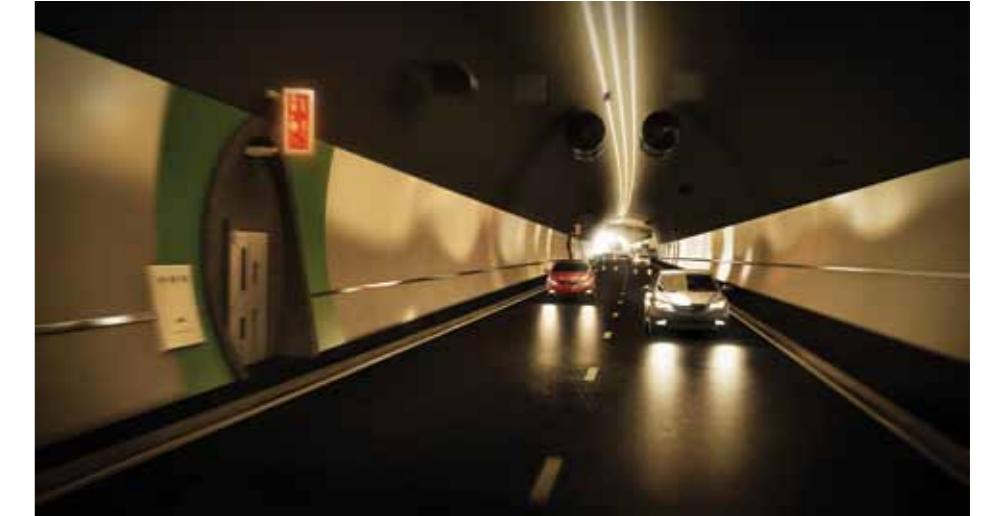
Figure 6.13: View of the inside of the tunnel
