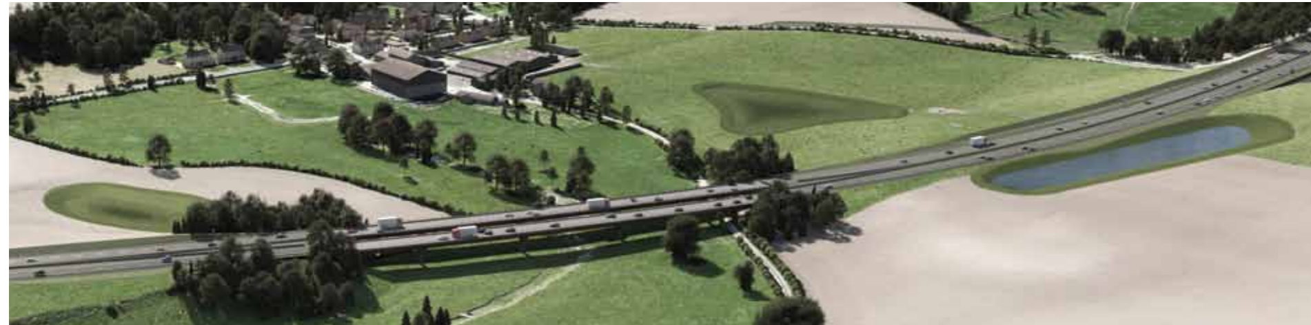
22 Figure 5.12: Road drainage infiltration areas either side of the River Till
