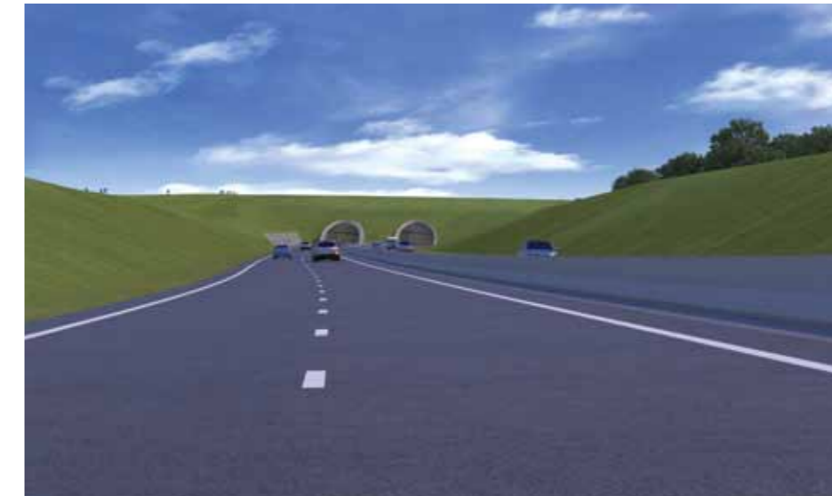
Figure 5.29: Driver's view of western tunnel entrance - grassed slopes option
