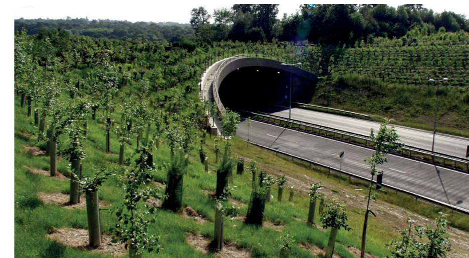
An example of a green bridge
