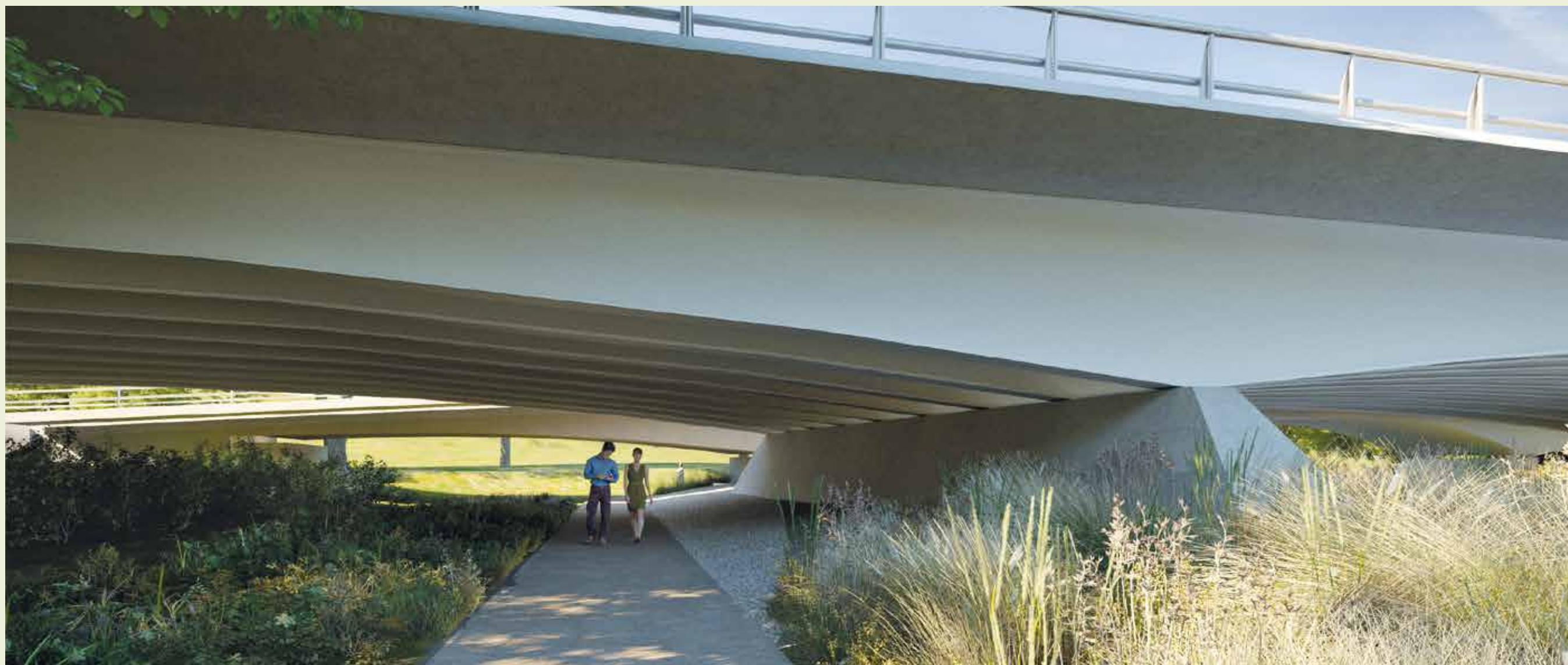
Throughabout Beige (Option 1V9) – Divides the existing roundabout in two. The lower bridge deck will produce a very restricted ground condition and may also create an intimidating space for users.
