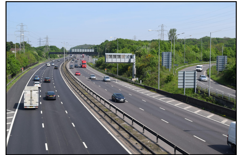
VP3: B255 bridge over A2: looking east along the A2
