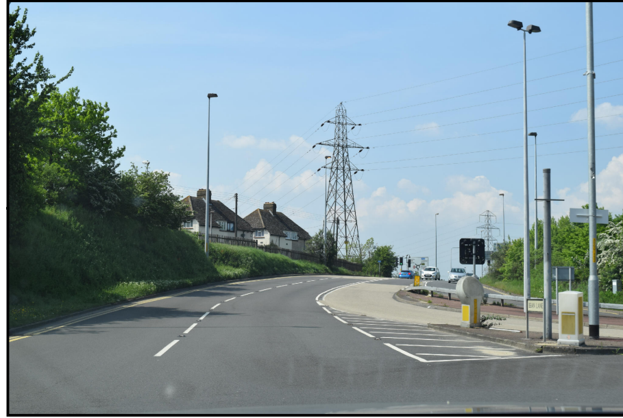
VP14: Roundabout south of Bean Junction: View looking north towards Bean Junction, on the left Hope Cottages
