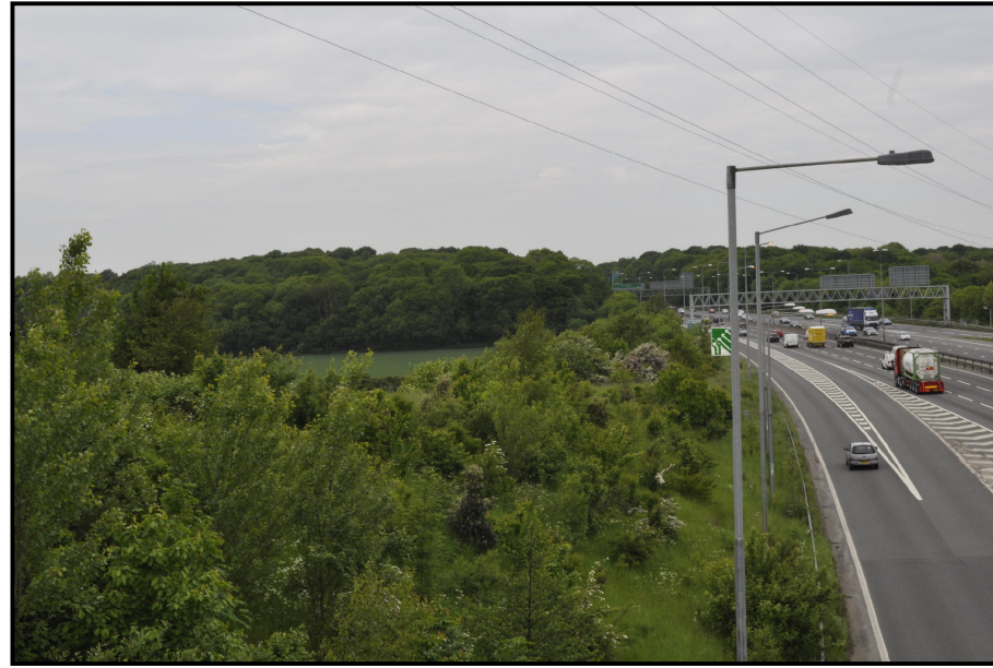
VP2: B255 bridge over A2: looking west along the A2
