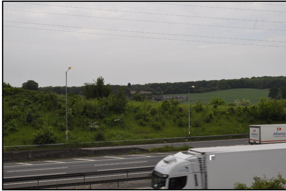
VP13: B255 bridge over A2: looking southwest towards Bean Farm (Listed Building)
