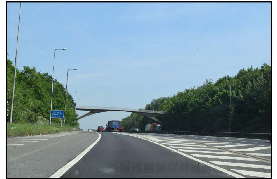
VP6: A296, Roman Road: View looking east, end of sliproad towards the A2
