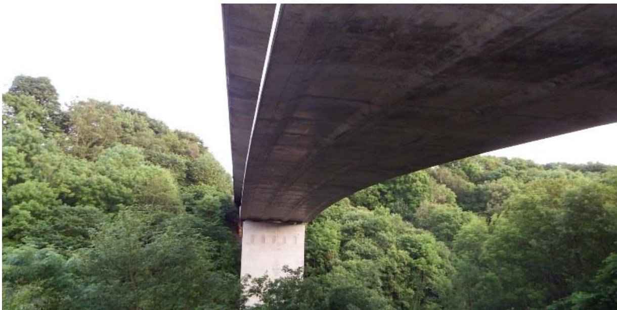
Image 7 - Existing River Coquet Bridge (looking south towards Ancient Woodland)
