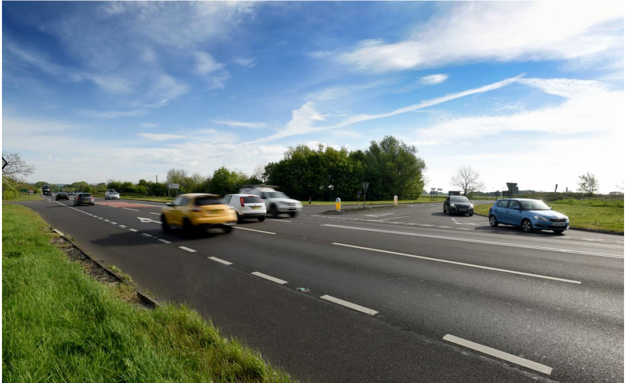
Image 6 - Existing junction at West Moor
