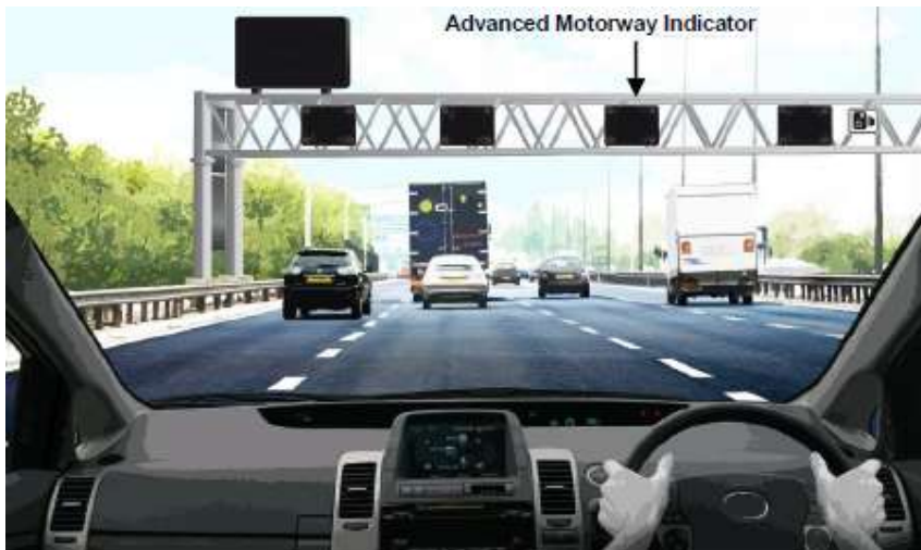
Figure 4a: Illustrative smart motorway scheme section operating in normal motorway conditions with blank advanced motorway indicators and blank gantry mounted variable message sign
