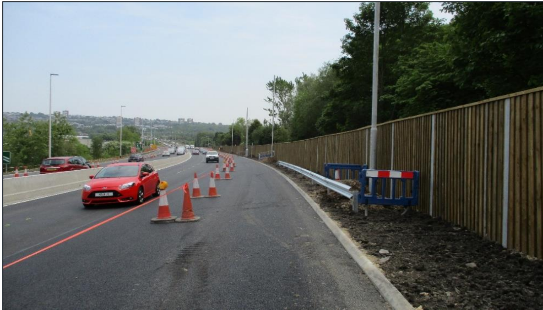
Photograph 6-6 - Existing Noise Barrier at along Lady Park adjacent to the A1
