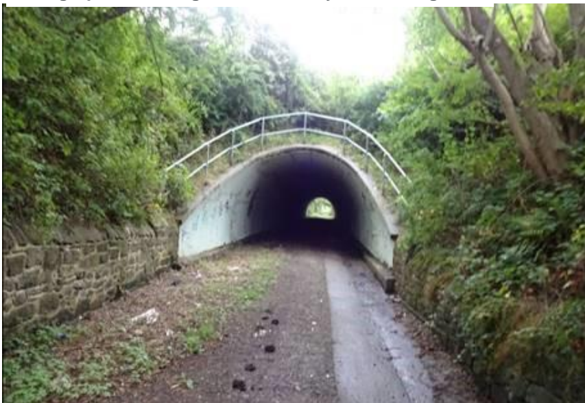
Photograph 6-1 - Longbank Bridleway Underbridge
